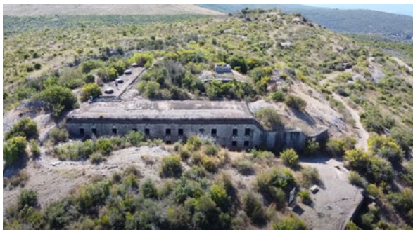
Figure 7 The current condition of the Traste Fortress – illustrating neglect and physical decay as forms of silent heritage. Source: dneвно.me, accessed August 28, 2025.
