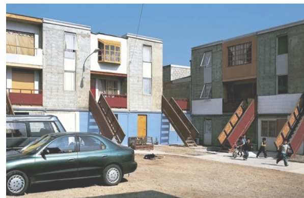
Figure 5a Elemental's Quinta Monroy housing – original façade. "Half a House" concept. Original units built by Elemental. Source: Cristobal Palma, 2006.; 5b Expansions to the original units completed by the residents. Source: Cristobal Palma, 2006.
